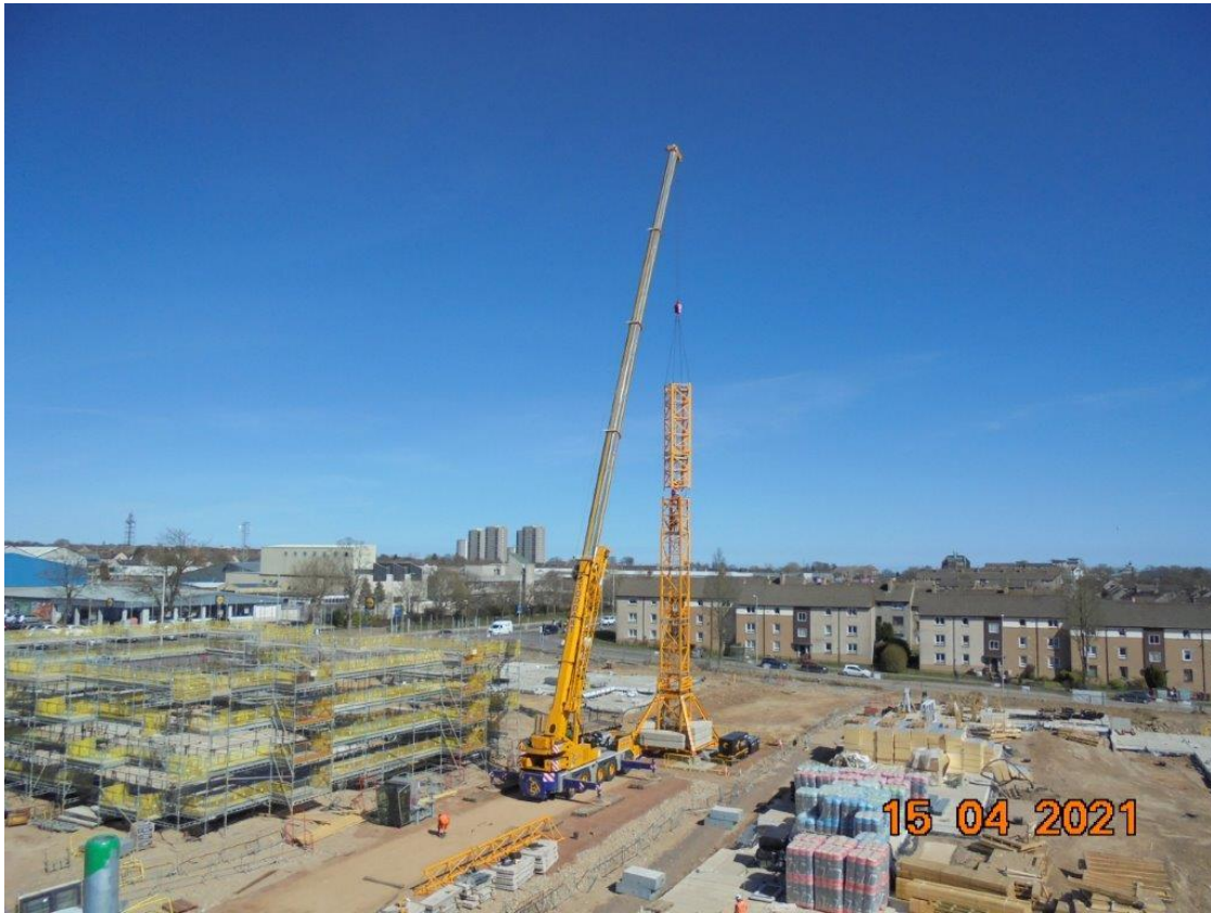
Block 3 – Scaffold and tower crane erection (15.04.2021)
